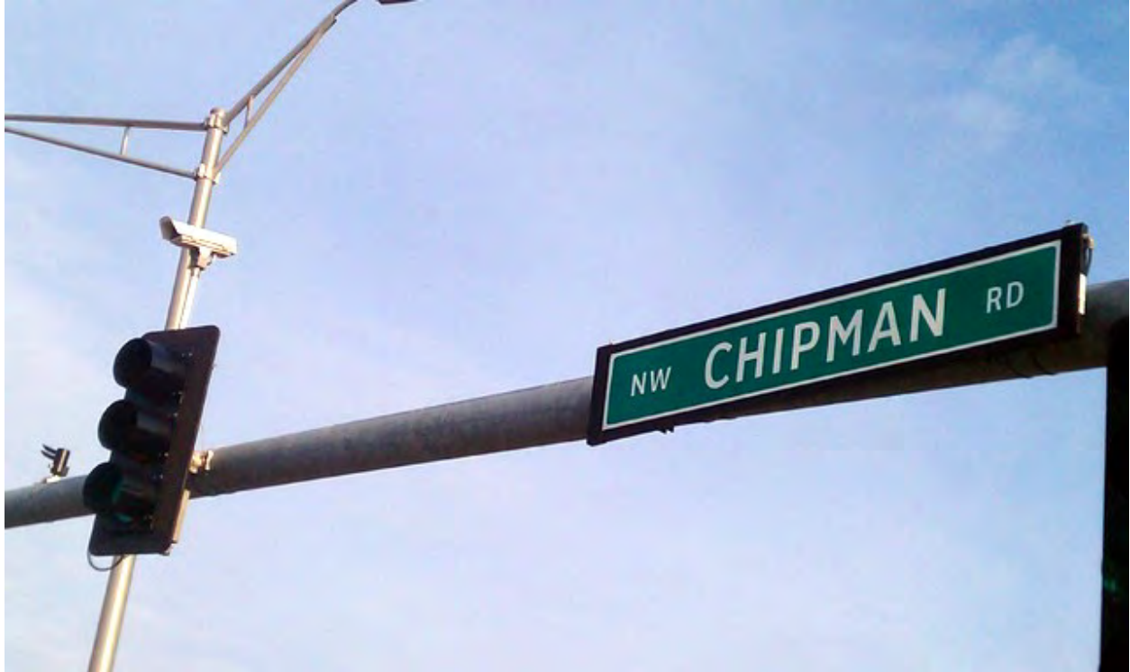
A mast arm on Chipman Rd. with mounted IP video camera for vehicle detection.
