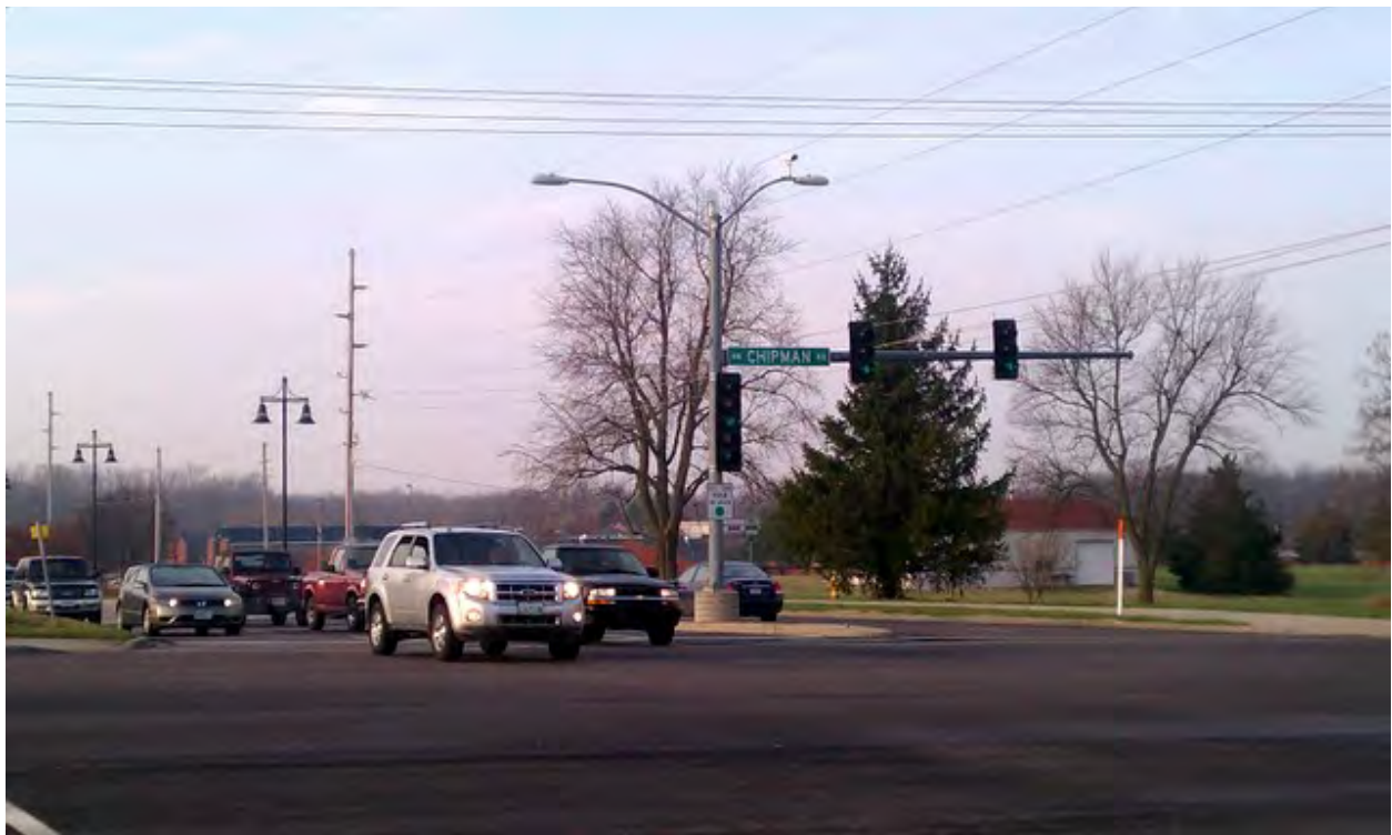
The InSync system installed on these traffic signals allows motorists to move through busy corridors without stopping. This saves time, fuel and frustration.
